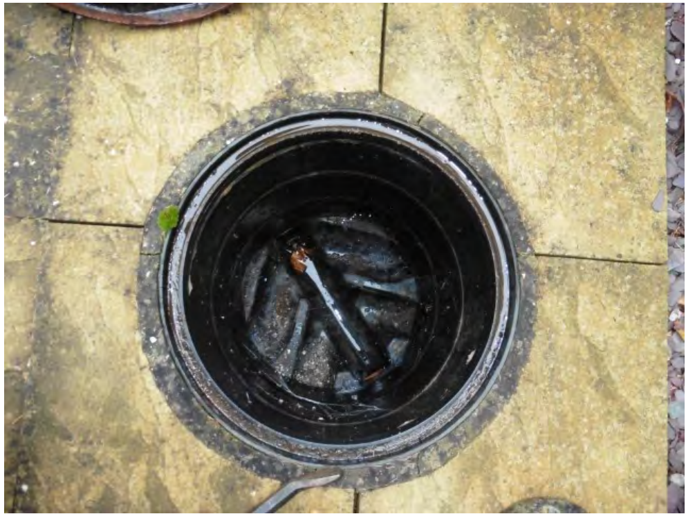
Inspection chamber to the front
