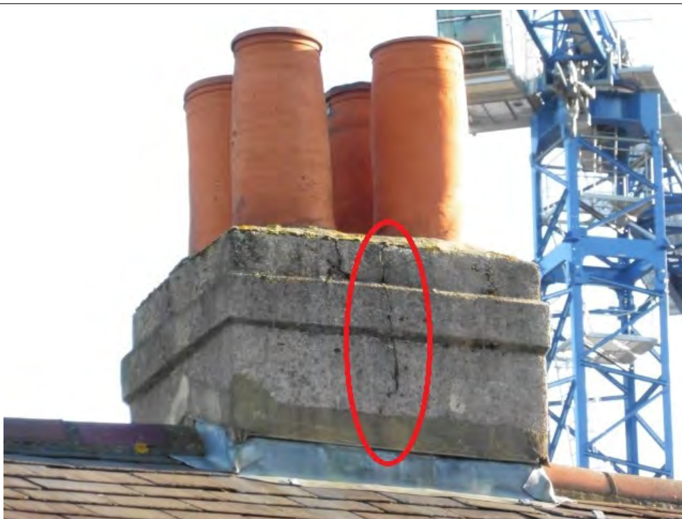
Central stack viewed from the front
